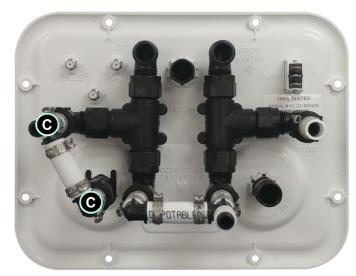
To connect pressure from pump plumbing harness, screw swivel fittings onto diverter valves (WATER INLET & FROM WATER) • as illustrated. This line will run directly to "OUT" side of water pump.
